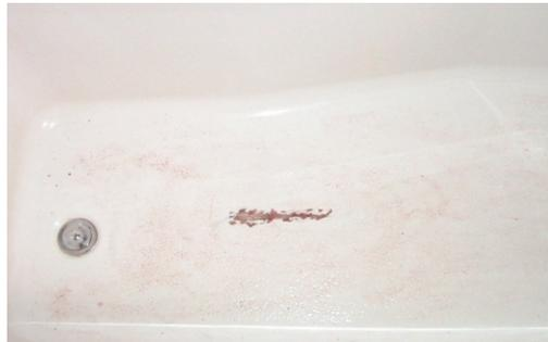
Original tub shower bottom worn, stained and cracked
